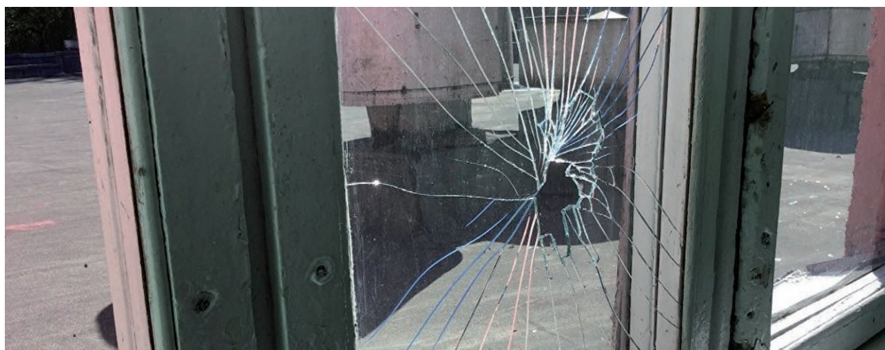
Fig 2. General view of radial cracks formed when glass fixed in the frame is broken.
