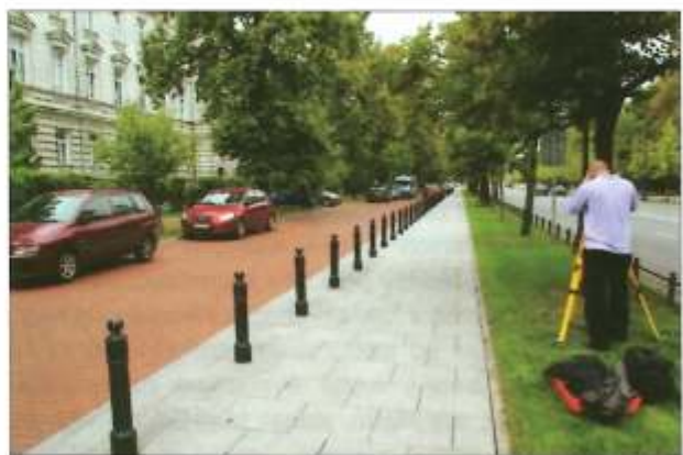
Ryc. 35. Pomiar jezdni z pasa zieleni Fig. 35. Measurement of road taken from lawn
