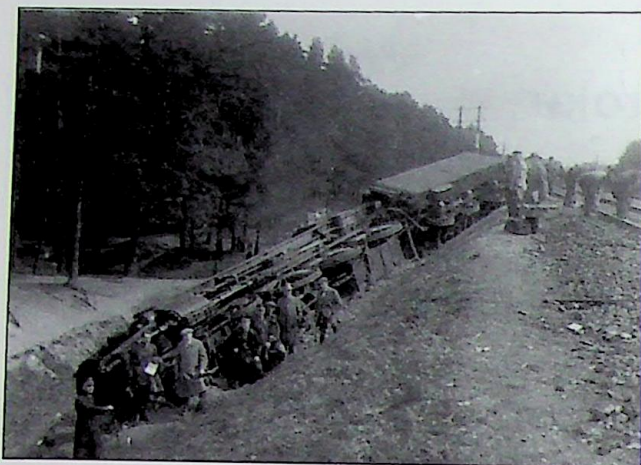
Ryc. 3. Wywrócona maszyna od strony nasypu z przodu Fig. 3. Overturned railway engine, front view from the embankment
